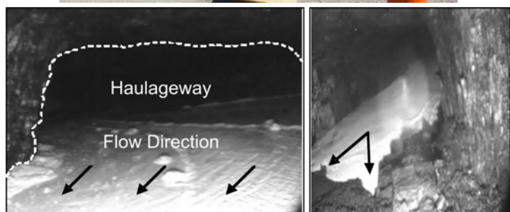
Video Image during Foamed-Sand Backfilling
